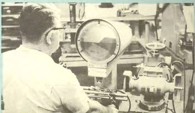
Comparator, used in making or repairing precision tools.
